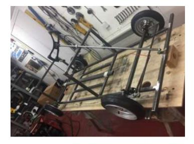
Fit front steering components, hubs, wheels, steering rods, steering column.
