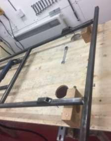
Temporary bolt front axle blocks to the chassis. Fit pre made front axle, as per drawing, to axle blocks, ensuring all measurements are correct and equal, and axle is square to chassis, weld in place.
